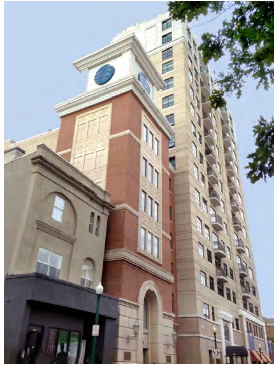
TCC District Building
