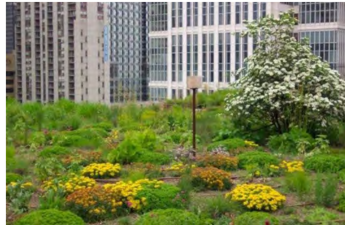
Intensive Green Roof
